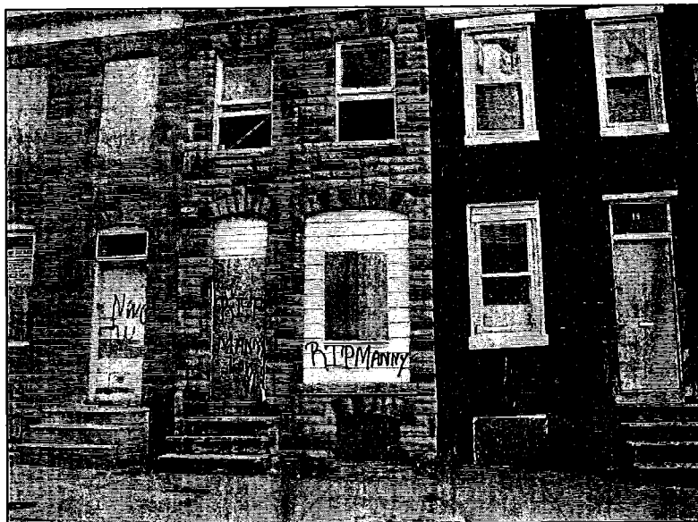
Figure 6: Boarded-up vacant houses are a problem.
