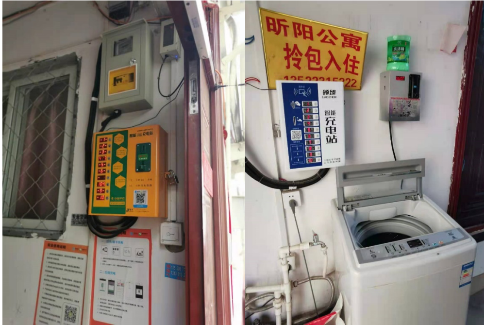
Fig 2. Charging stations by apartment entrances where residents can prepay for electricity.
