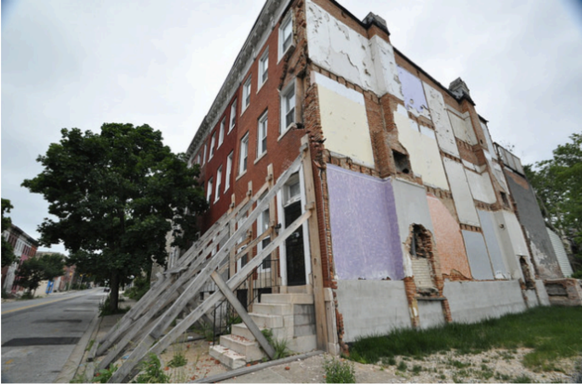
Figure 28: Occupied row house incurring damage because of destabilized wall from demolition of neighboring house, 2016.
