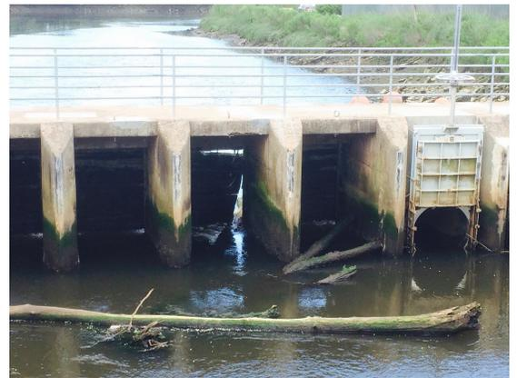
Figure 11: Examples of large debris in SRTG (left) and traditional wooden flap tide gates (right) during study period. While these issues complicated monitoring at the site, they were often resolved through regular tidal flushing or coordinated removal with the City of New Haven Engineering Department.
