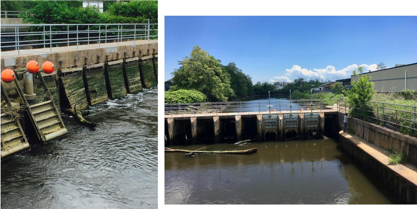
Figure 4: SRTG system on the West River – Left photo shows perspective on downstream (harbor side) of SRTG (i.e. those with orange floats) and traditional wooden flap tide gates. Right photo shows perspective on upstream (river side) of SRTG. Blue gate valves on right side of photo show means of manually closing SRTG (photo credit: Laura Green)
