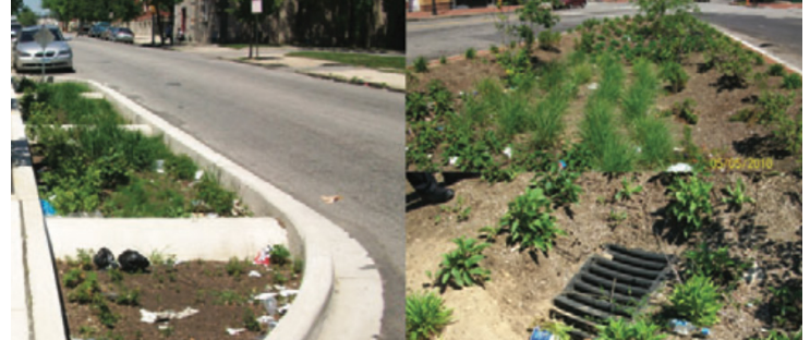
In Baltimore , 12 bio-infiltration basins were installed in a subwatershed. After 4 years, a study found a 50% reduction in nitrogen and phosphorous in the basin's stormwater samples
