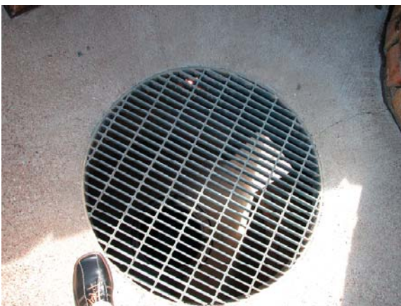
View through top floor grate to first floor.
