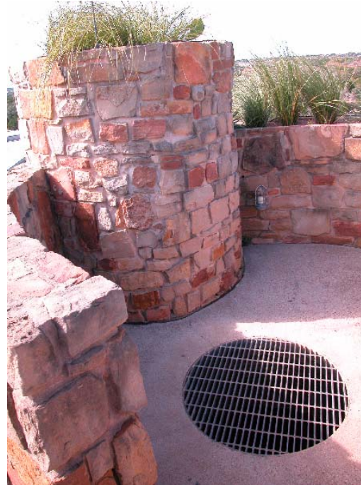
The top floor is graded to drain all rain through this grate.
