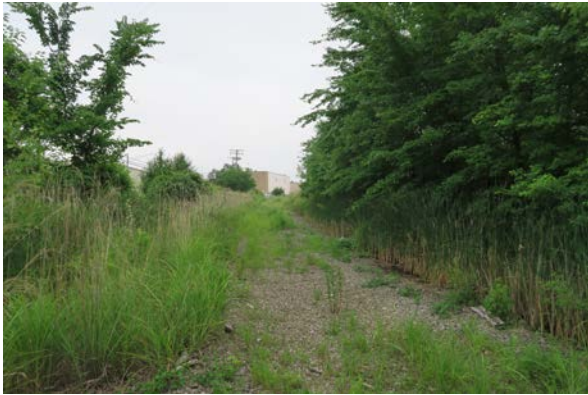
Morrell Park (Abandoned CSX tracks)
