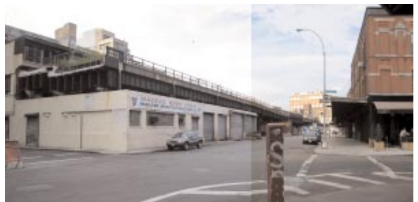
Fig.9: - End of demolition at Gansevoort Street
