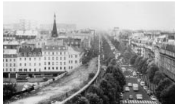
Fig.5: Aerial view of the Viaduct Daumesnil
