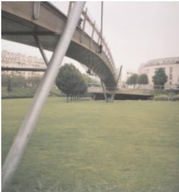
Fig.18: The bridge at the Promenade Plantée
