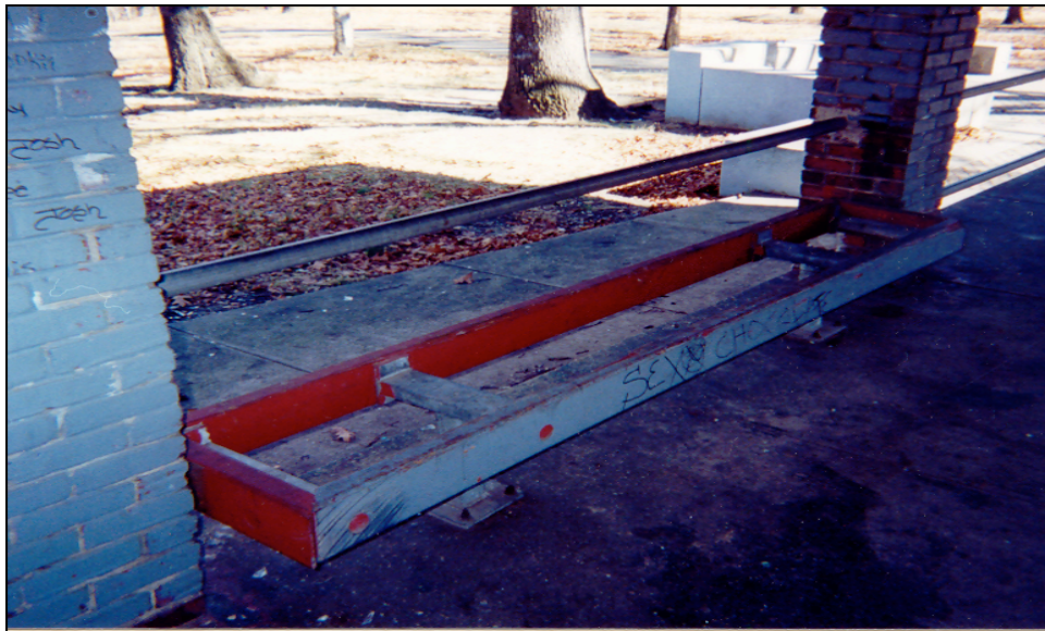
Figure 23. A closer examination reveals that the pavilion is dilapidated. Carpenter. February 2002.
