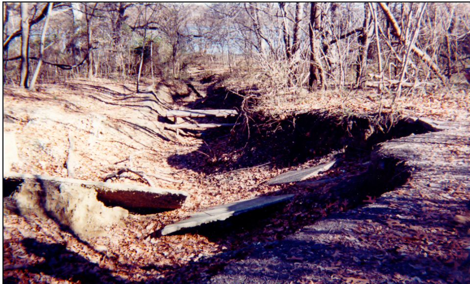
Figure 17. This area of severe erosion can be found perpendicular to a nature trail in the park (see previous figure). The broken concrete pathway in the eroded area is the nature trail. Towards the center of the photo, a picnic table is visible which serves as a makeshift bridge for the wanderers in this area of the park. Carpenter. February 2002.
