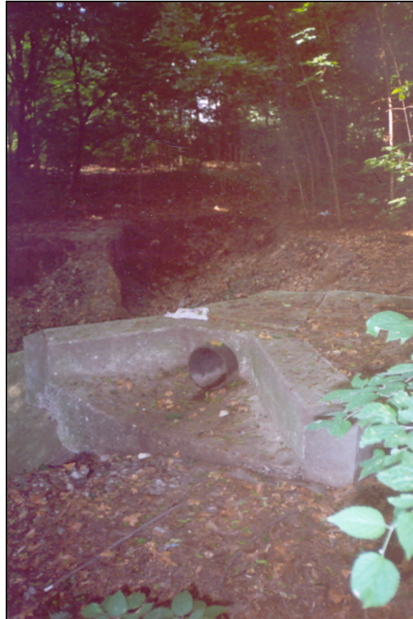
Figure 10. This storm water drain is exacerbating erosion on the escarpment. I submitted a grant application for the installation of a storm water drainage system on this area of the escarpment. Carpenter. August 2002.
