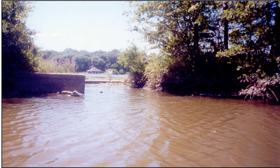
Figure 12. Facing the park, this area shows a smaller break in the dike. This rupture is about five feet wide. Carpenter. August 2002.
