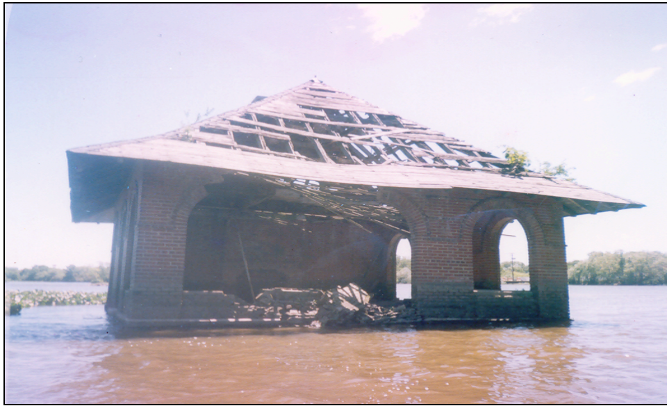
Figure 14. Once an edifice used for picnicking and socializing, with a beautiful view of the meadow, this edifice now stands in ruins in the flooded area of Farnham Park. Carpenter. August 2002.
