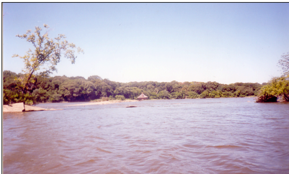
Figure 11. Facing the park, this area shows the major break in the dike that occurred in 1971. The rupture in the dike is approximately forty feet wide. Carpenter. August 2002.
