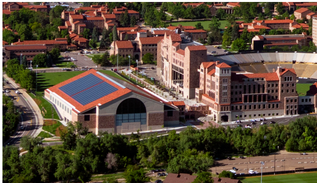
An 850-kilowatt solar array tops the Indoor Practice Facility next to Folsom Field on CU Boulder's Main Campus. Photo by: Glenn Asakawa/University of Colorado Boulder
