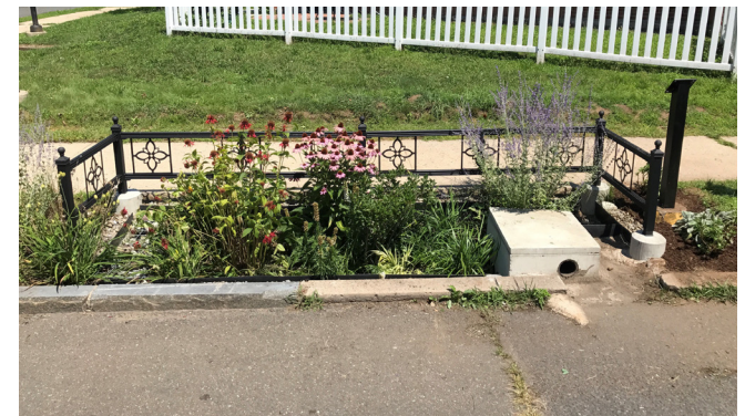
Bioswale with device to monitor volume of stormwater capture.
